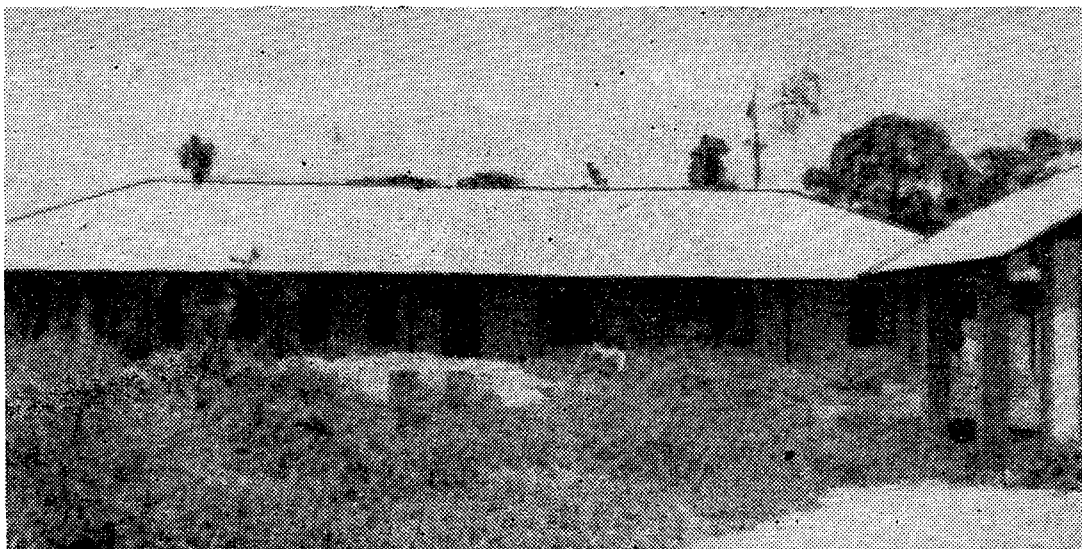
The first ward of the new Nigerian hospital. Part of the operating room can also be seen on the right of the picture.
